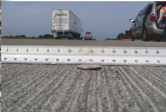
The pavement on the left was finished by the artificial-turf-drag method, and the pavement on the right has been both diamond ground and grooved.
